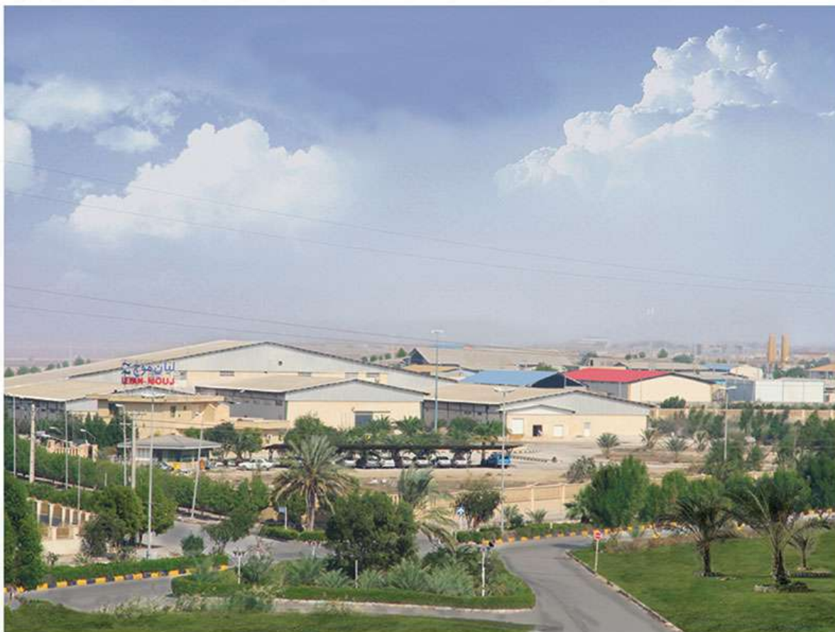
Bushehr Industrial Park
